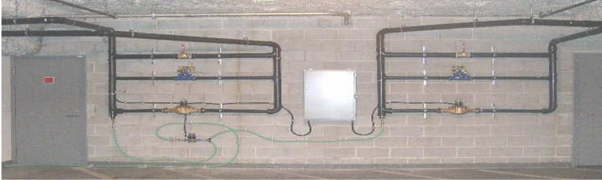
A pressure relief valve was installed in parallel with the water meter, and will open if the meter becomes fouled. A bypass valve was also installed as an additional redundant measure. To date, both the bypass valve and pressure relief valve have not been used. However, debris does accumulate on the meter strainers. The 50mm strainers are cleaned every three months and the 19mm strainer every 2 weeks.
