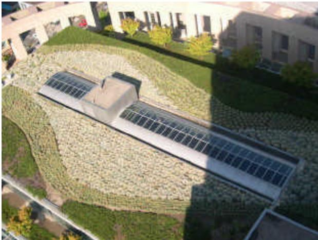
The Vancouver Public Library's (VPL) Central Branch building and green roof were constructed in 1995. The 2,600 m<sup>2</sup> (28,000 sq.ft.) roof includes an extensive green roof with a gross area of 1850 m<sup>2</sup> (20,000 sq.ft.) and a net area of 1,500 m<sup>2</sup> (16,150 sq.ft.). The green roof was designed and completed by architect Moshe Safdie and Landscape Architect Cornelia Hahn Oberlander.
